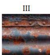
Rusting of Iron
